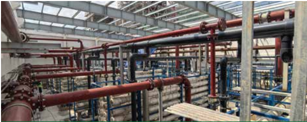
Green Hydrogen Demonstration Project Material Procurement
