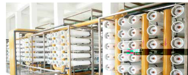
Xilinhote Municipal Water Plant
